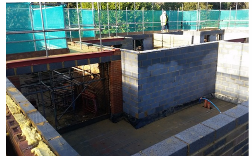
Brick and block work to first floor - 13/01/2015
