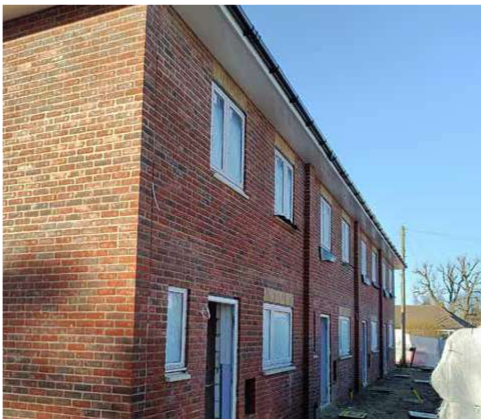
Our two bedroom flats at Beynon Court , Warlingham nearing completion.
