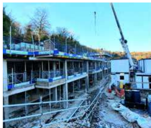
Construction ongoing at Bronzeoak House .
